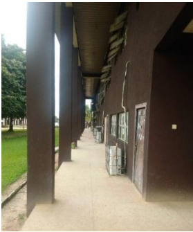
Figure 1 Open Corridor (Long Hallway)
