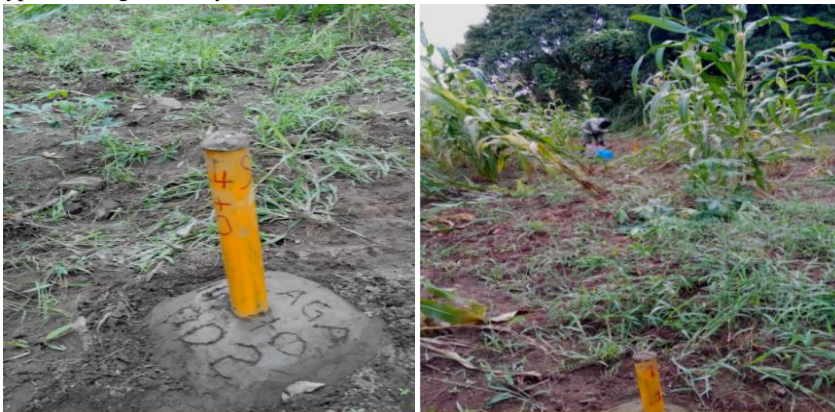
Figure 6: The Pegging of a Tower Center Point and its Offset Points
