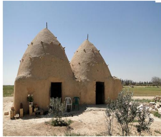
Figure2: A picture showing a typical Nigeria mud house with dome roof
