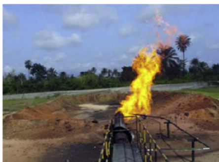
Fig. 2: Gas Flaring at onshore field location in Rumuekpe, Rivers State.
