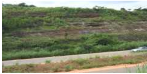
Figure 4: showing overview of the exposed section in Umunya, about 18km from Onitsha along the Enugu-Onitsha Expressway
