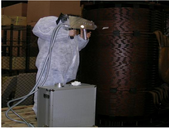
Figure 5: A field assessment of transformer condition using TRANSPEC™ (Source: [18])
