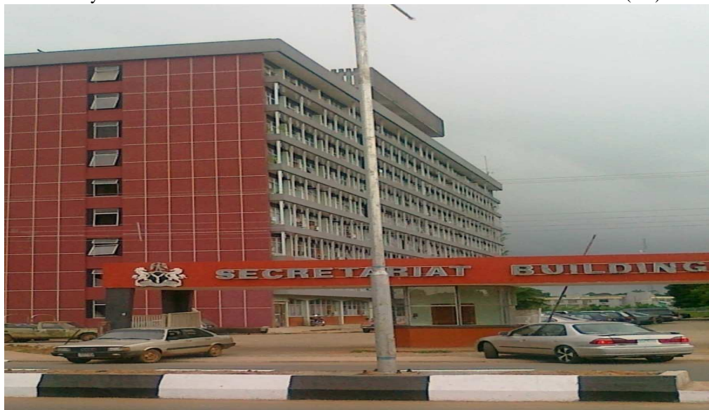
Figure 1: Secretariat building Sapele road, Benin City, Edo State, Nigeria.
