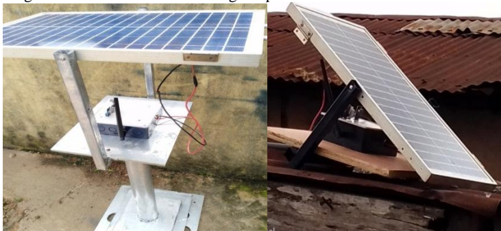
Fig 12 Completed and installed WSN nodes on site; sidewalk and roof top
